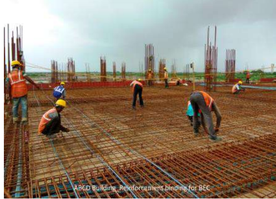
Reinforcement for BEC Slab
