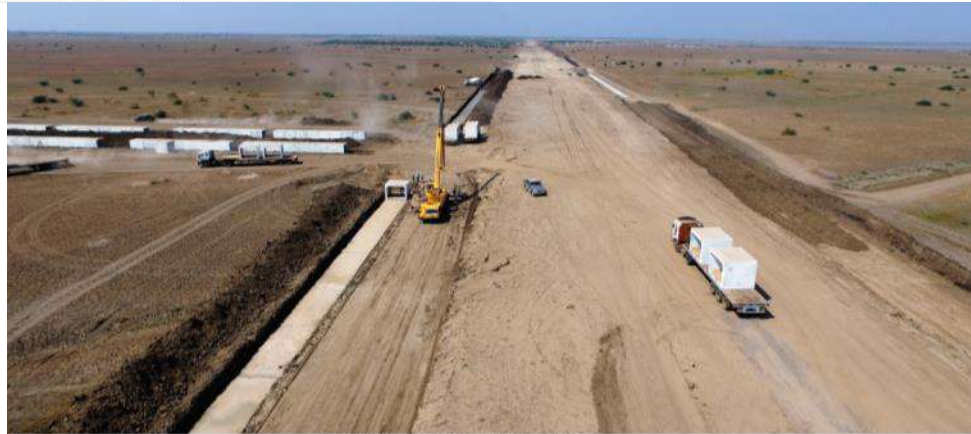
Power Duct Laying In Progress. - H-1
